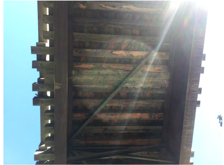
Deck from underneath
