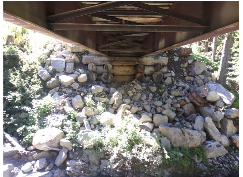
Left Bank Abutment when facing downstream
