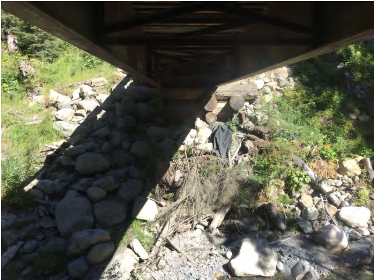
Right Bank Abutment when facing downstream
